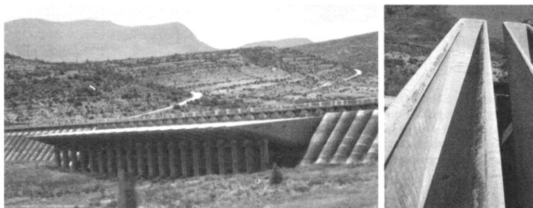
Figure 1. Beni Bahdel labyrinth spillway upstream view (left) and top view (right).
